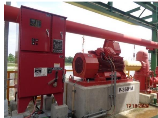
Electrical Driven Fire Water Pump
