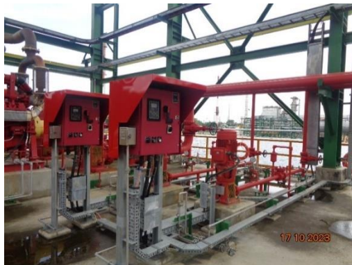
Electric Motor Driven Jockey Pumps
